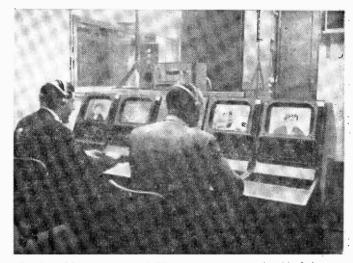
The first of four Marconi Mark IV television cameras ordered by Independent Television News is now in use at the I.T.N. headquarters in London. By November all four cameras will be fully operational in a new studio which is being built on the seventh floor. This picture shows the I.T.N. control room, with the control desk for the cameras.
