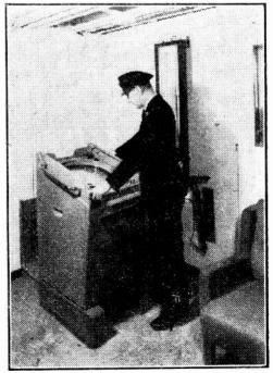
The new Orient liner, "Orsova," is the first ship to have the new Marconi Marine 15in. "Radiolocator" radar. One of the "Orsova's" navigating officers is seen watching the screen of the new radar in the liner's chartroom.
