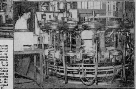
The above illustration shows the completed bulb being removed from the machine by means of a 'acuum chuck. When the chuck is not in use, it is housed in a box held at the same temperature as the finished bulb. On the right is the glass parts joining machine, showing the necks and heads of the picture tubes clamped
