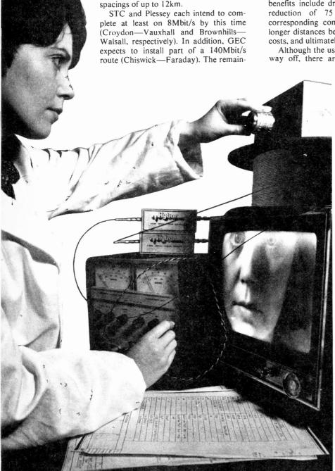
A video camera connected via a fibre optic link to a monitor. The reel holding the fibre optic element and the modems can be clearly seen. (Pilkington Ltd.)
