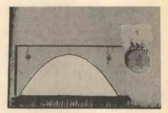
Parabolic groove in lid to take top of reflector
