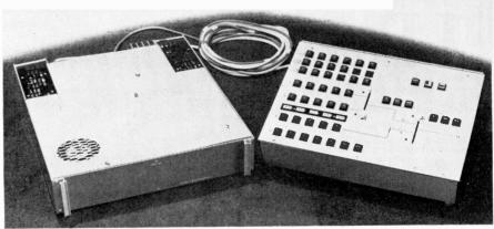
Experimental digital vision mixer developed by the IBA. Input and output signals are coded in linear PCM, at a sampling rate of 2fsc. The mixer offers additive mixing and split-screen wipe facilities
