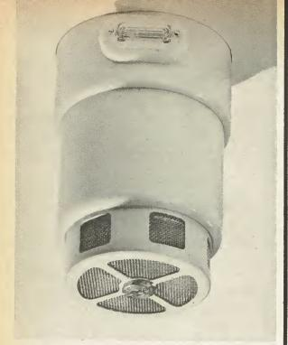
The Minerva ionisation chamber smoke detector. This unit is mounted on the ceiling and gives early warning of fire. A trigger tube is employed to operate a relay
