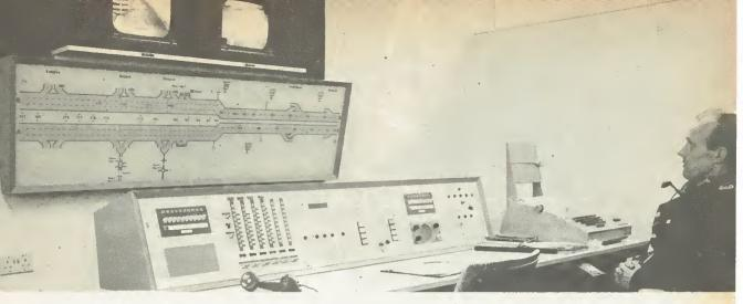
Control centre for M4 Signalling System showing the control desk, mimic diagram and closed circuit television monitors. Situated on the desk is the control for emergency telephones, police radio and closed circuit television
