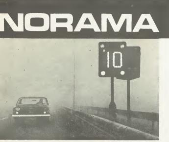
Post mounted signal situated on the central reservation, showing 10 m.p.h. speed restriction
