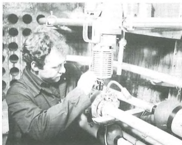
FIG. 11—Injection welding of sheath closure in progress
