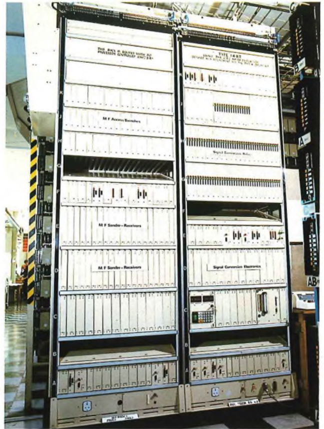
FIG. 4—Type 14 register-translator (1980)
