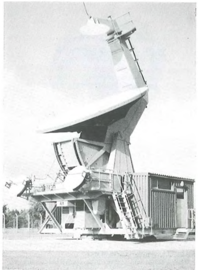
FIG. 10—The Martlesham 6 m diameter steerable aerial
