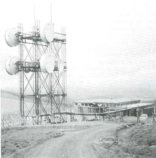
FIG. 15—Tower No. 5A
