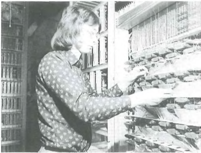
FIG. 8—TXE4RD cyclic-store data-threading field (1976)
