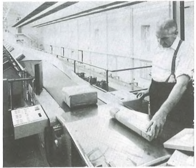
FIG. 1—Tilted-belt parcel sorting machine
