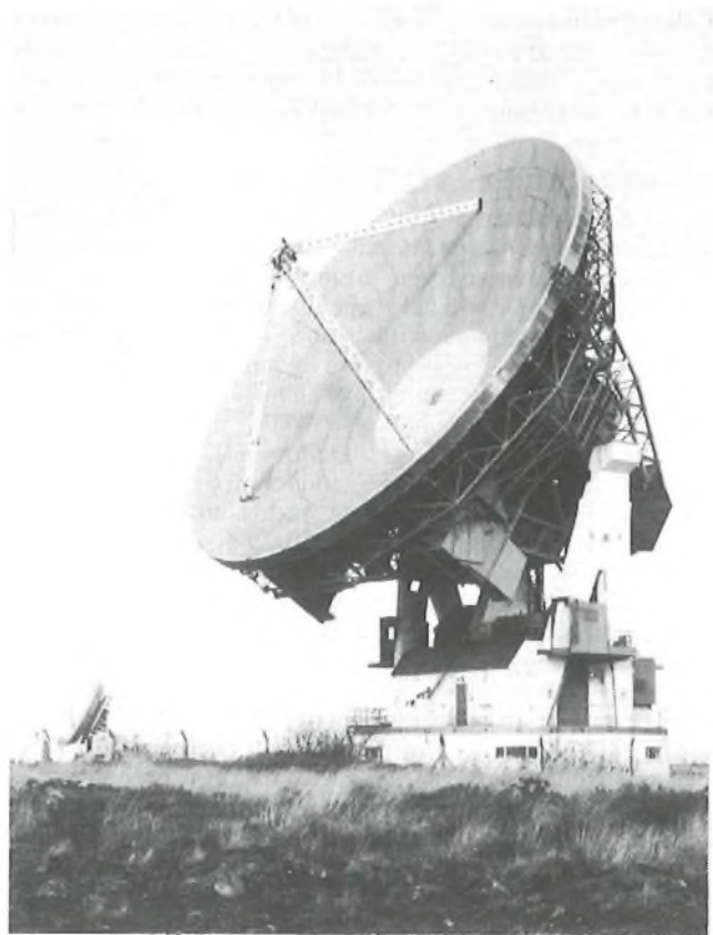
FIG. 2—The Goonhilly 1 aerial, Goonhilly Downs, Cornwall
