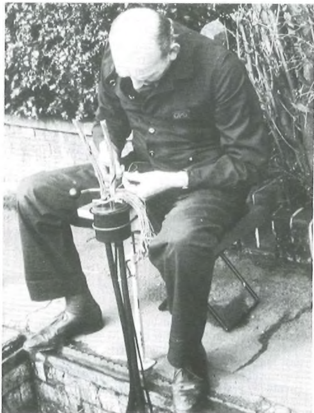
FIG. 9—Sleeve No. 31A with a jointing jig
