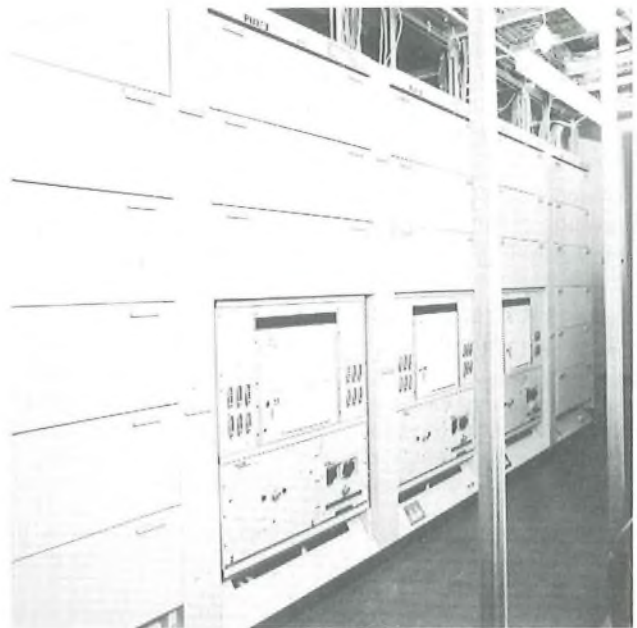
FIG. 9—System X large processor utility
