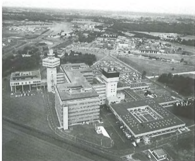
FIG. 1—Aerial view of the British Telecom Research Laboratories
