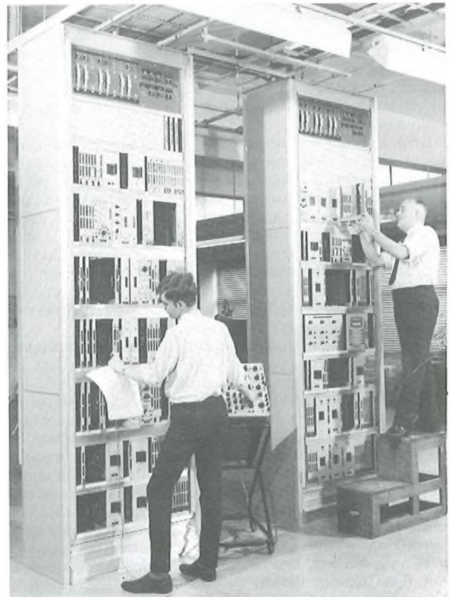
FIG. 2—The first PCM switching exchange in the world (Empress, London) used eighth bit in-channel signalling in 1968
