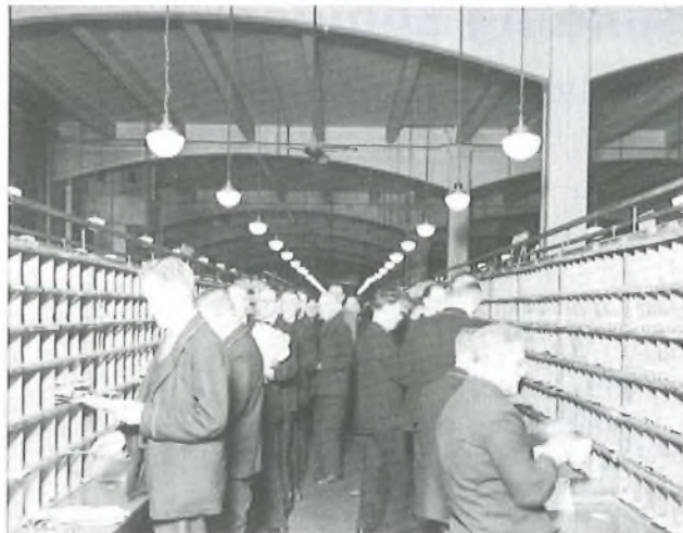
FIG. 2—Totally-enclosed filament lighting in use several years ago
