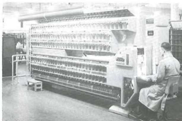
FIG. 2—Single-position letter-sorting machine
