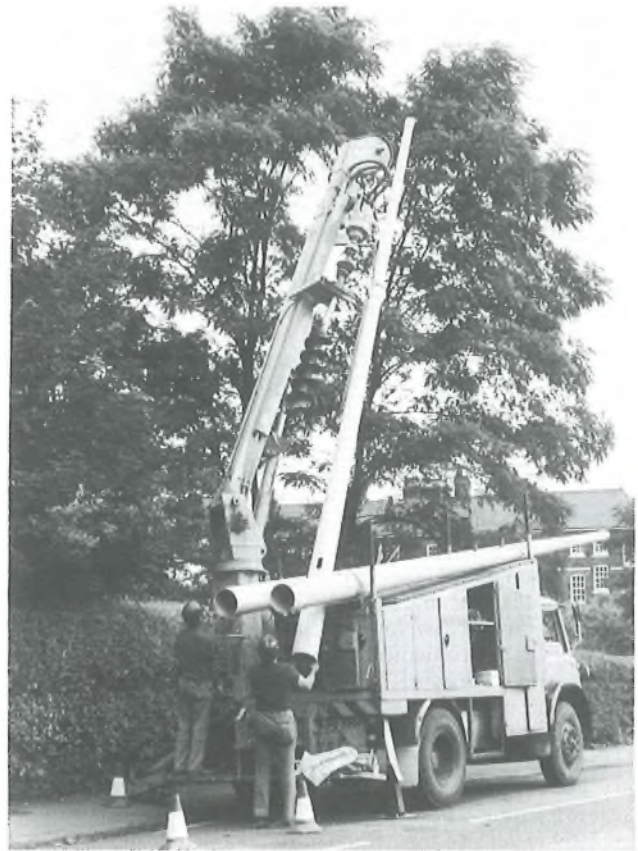
FIG. 13—Pole-Erection Unit erecting a hollow pole
