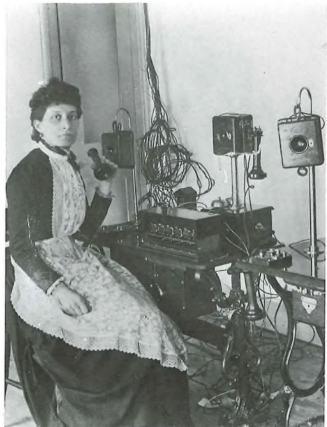
FIG. 2—The Blake microphone and the Bell earphone (In use at the Croydon telephone exchange in 1884)
