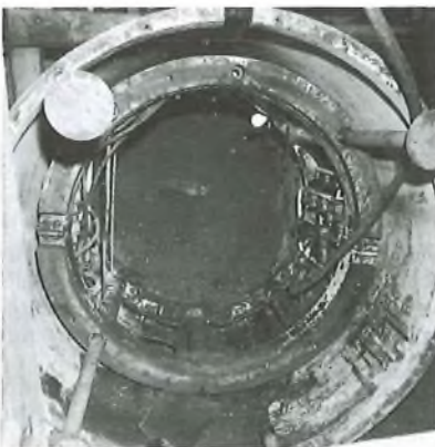
FIG. 2—Shield, showing driving rams
