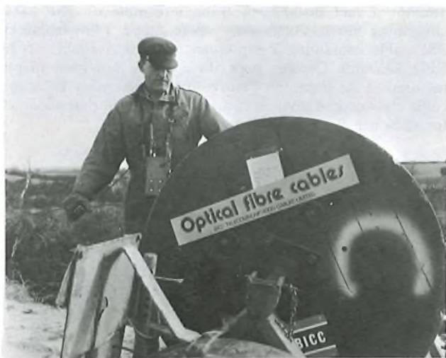
FIG. 4—Cable installation by Colchester Telephone Area staff
