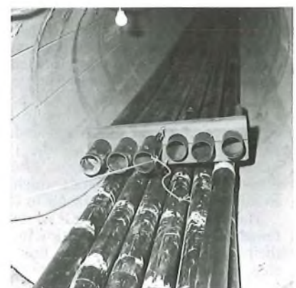
FIG. 4—The 6-way pulling clamp
