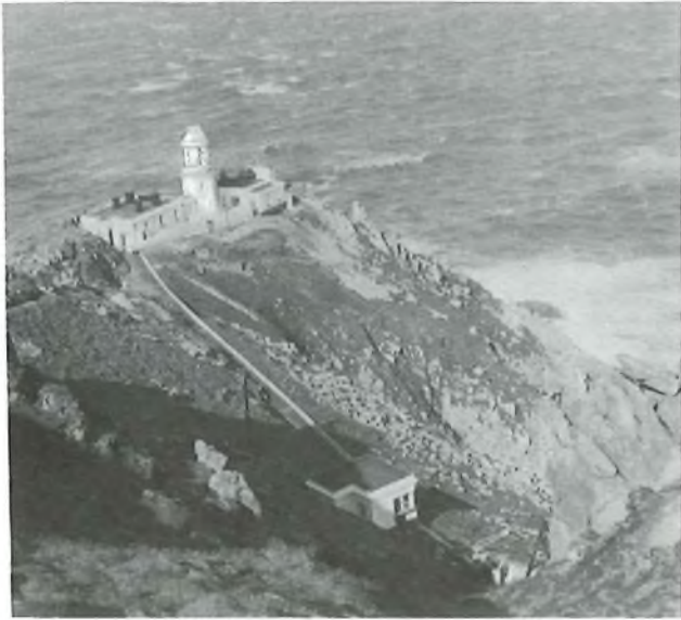
FIG. 3—The northern lighthouse
