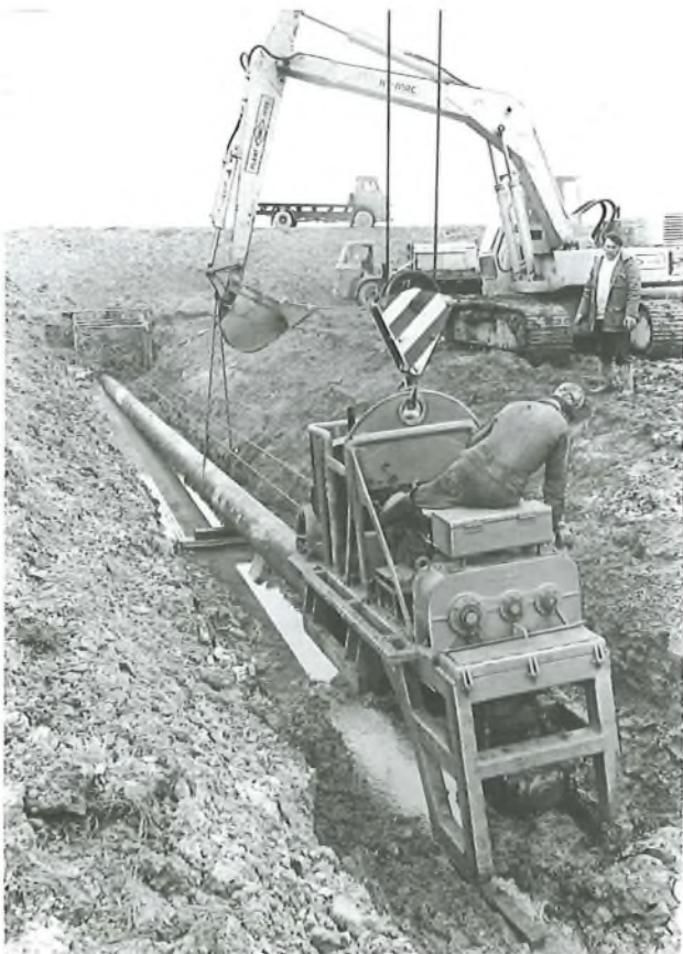
FIG. 2—The auger borer in operation
