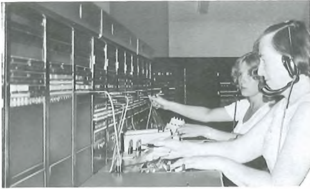
FIG. 2—Face panels at Braintree AMC after conversion
