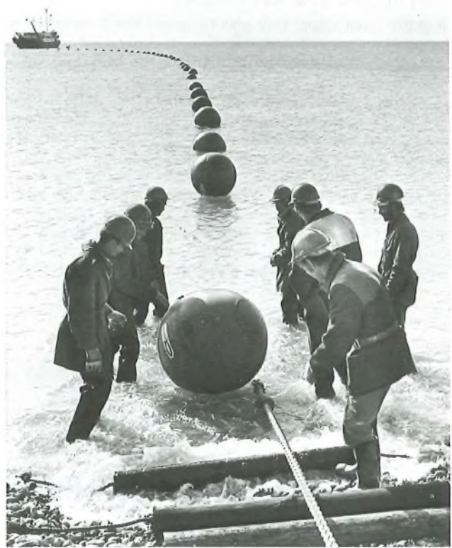
FIG. 4—Preparing to cut away the first float as the cable is brought ashore
