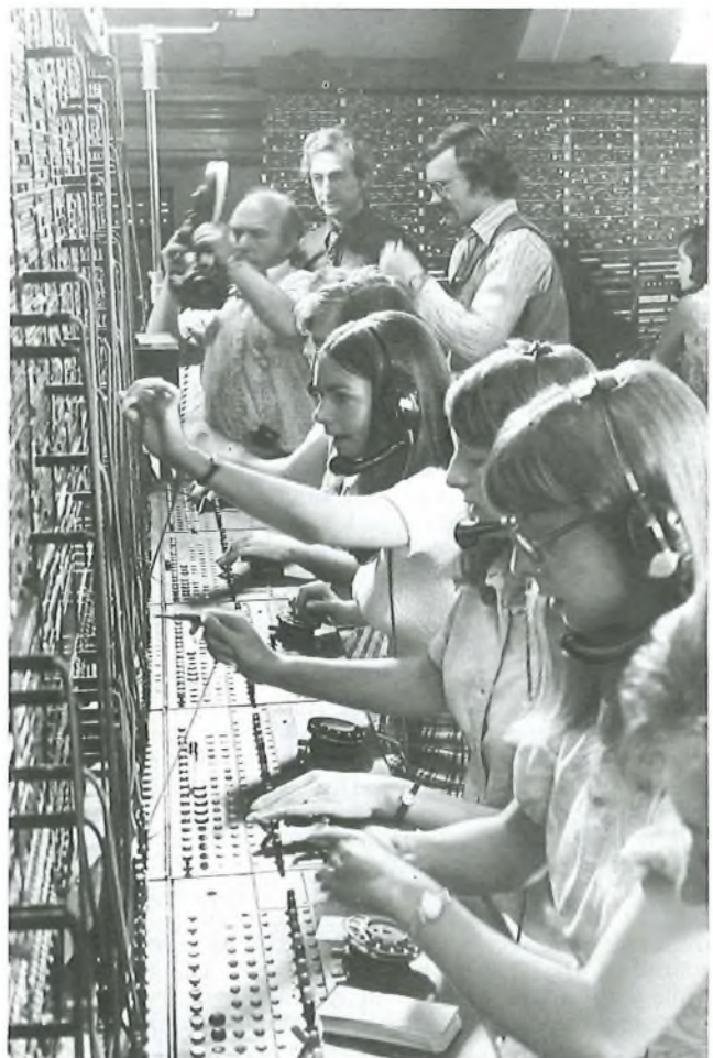
FIG. 1—Face panels at Braintree CB 10 before conversion
