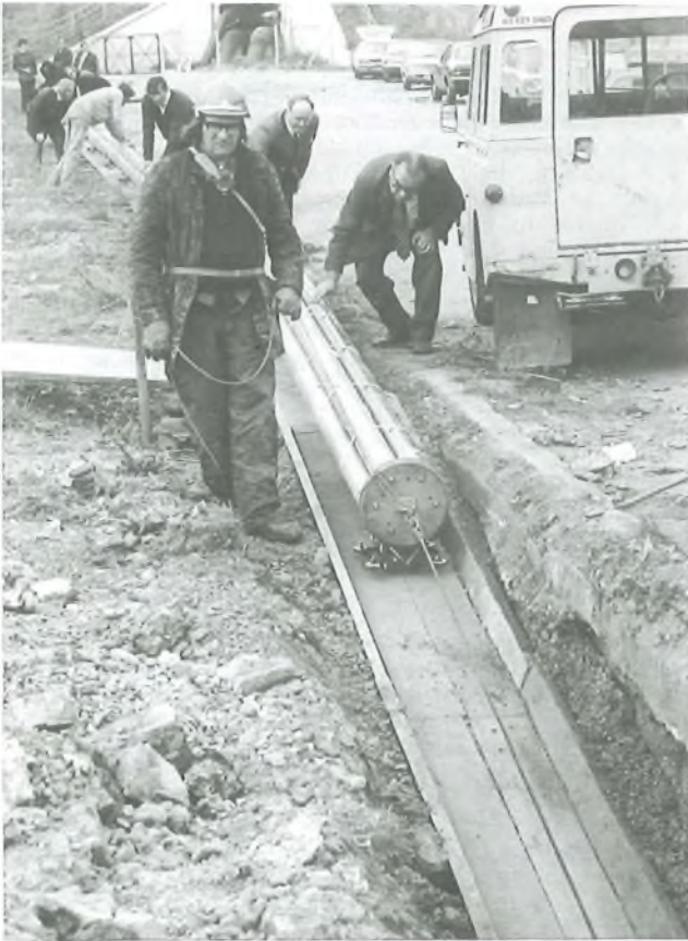
The assembled duct nest being drawn down the ramp to the gas pipe
