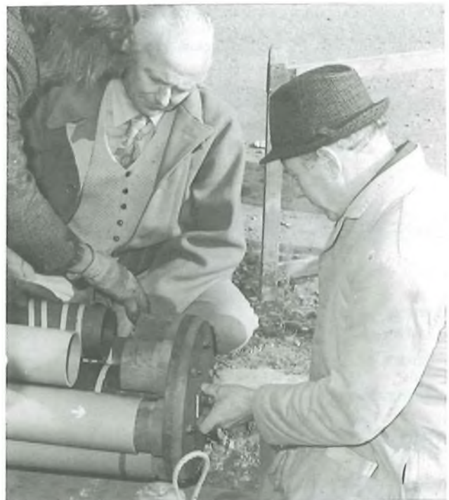
Fitting the front former to the ducts
