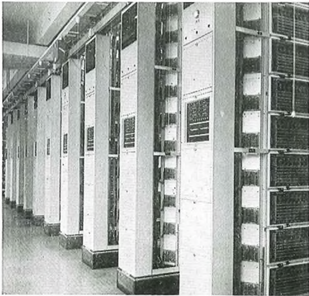
General view of Hastings TXK1 unit
