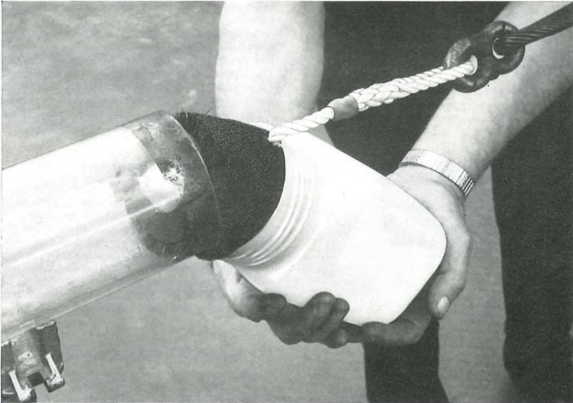
FIG. 5—Lubricating brush entering duct
