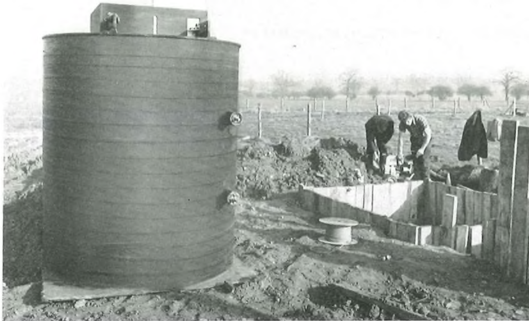
FIG. 4—The silo buried repeater station
