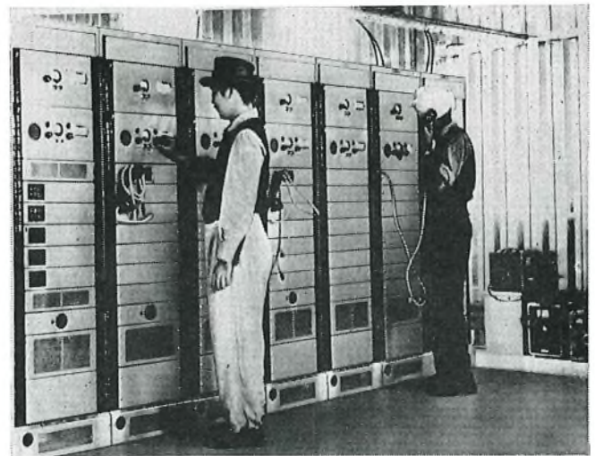
FIG. 6—FIVE-CIRCUIT JUNCTION RADIO EQUIPMENT INSTALLED IN NORTH BORNEO
