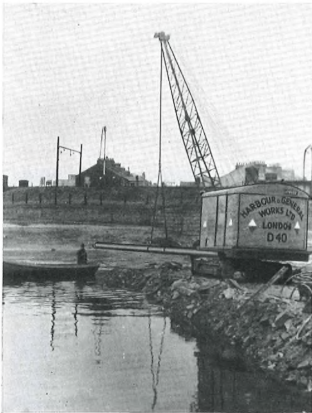
FIG. 2—THE DRAGLINE EXCAVATOR ON THE CAUSEWAY AT THE RIVER LUNE CROSSING
