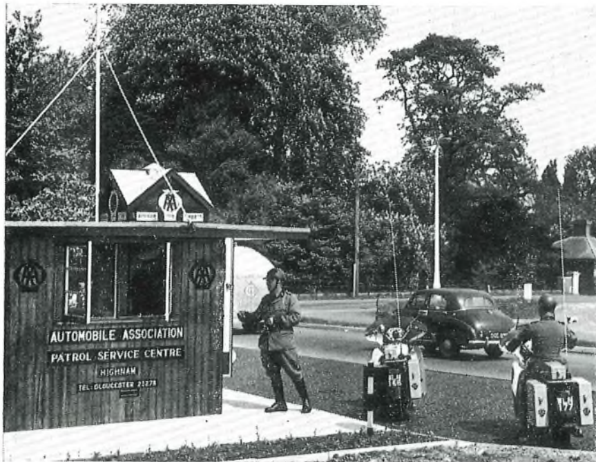
FIG. 1—TYPICAL MOBILE-RADIO-SERVICE BASE STATION
