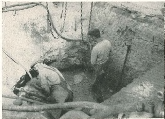
BREAKING UP THE OLD FOUNDATIONS
