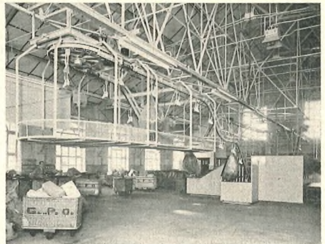
FIG. 2—DRIVE AND TENSION UNIT
