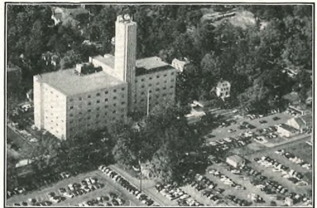
AERIAL VIEW OF THE WHITE PLAINS BUILDING, SOME 30 MILES NORTH OF NEW YORK CITY.
