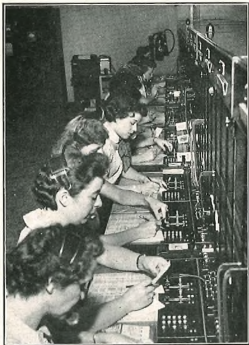
OVERSEA SWITCHBOARD IN WHITE PLAINS, NEW YORK, WHERE UNITED KINGDOM-UNITED STATES CIRCUITS TERMINATE.
