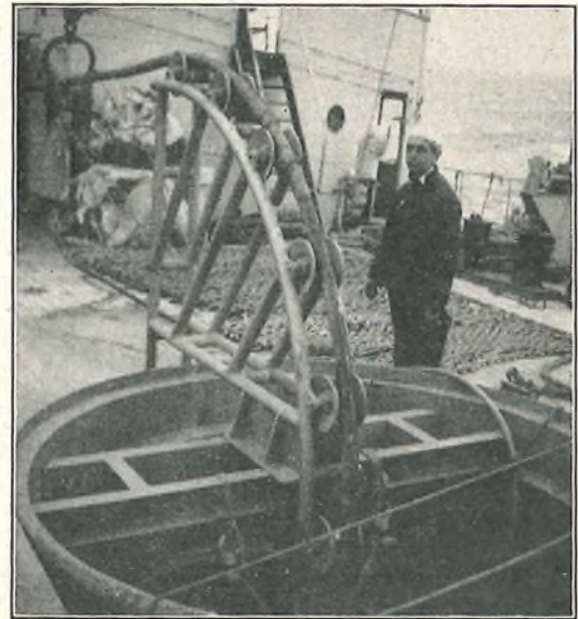
FIG. 7.—NEW ROLLER TRACK CABLE LEADS AT CABLE TANK NO. 1.
