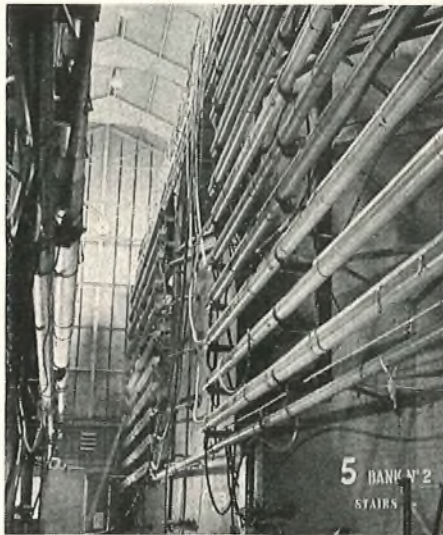
Storage tanks—each of which holds 200 miles of finished cable—showing troughs containing flexible repeaters spliced into the cable.
