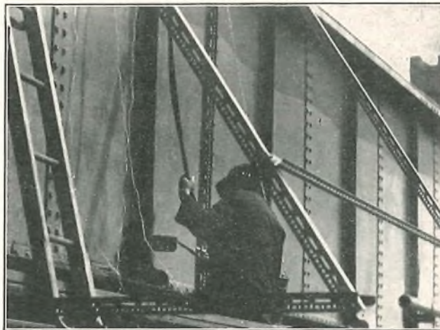
WELDER SUPPORTED BY DEXION FRAMEWORK ATTACHED TO BRIDGE ACROSS RIVER URE.
