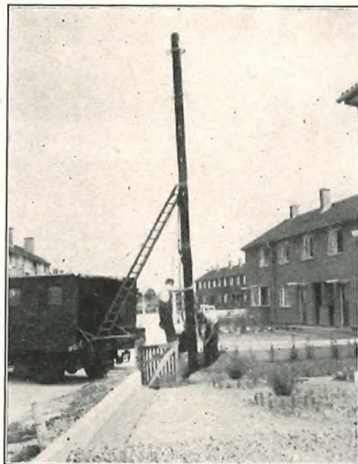
ERECTING A POLE WITH THE DERRICK.
