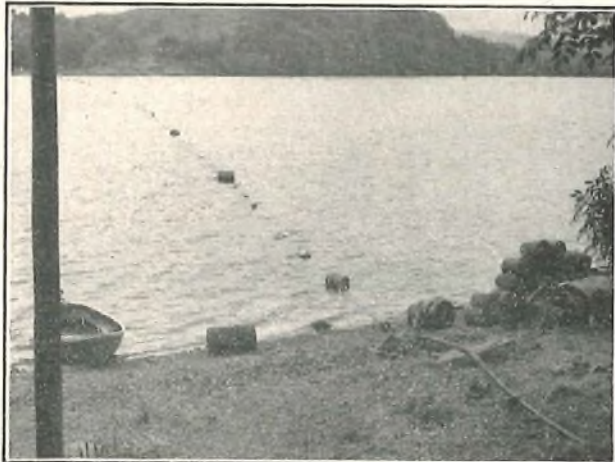
THE CABLE ACROSS LOCH AWE BEFORE STARTING TO PUNCTURE THE DRUMS.
