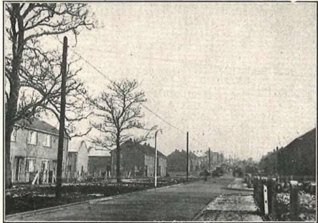
APPEARANCE OF TYPICAL AERIAL CABLE AND DROP-WIRE.
