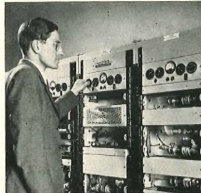
A rear view of the G.E.C. transmitting equipment at Cassel, relaying programmes to Swingate.
