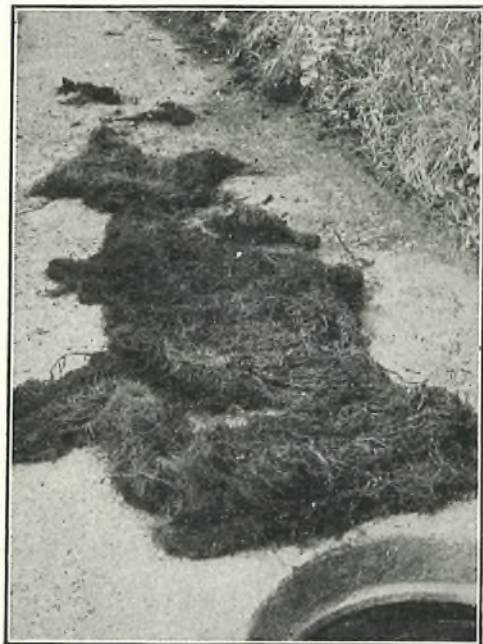
ROOTS REMOVED FROM MANHOLE.
