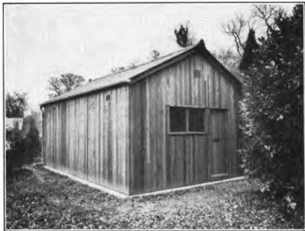
STANDARD B1 TIMBER U.A.X. BUILDING AT HEADLEY, NEAR EPSOM.
