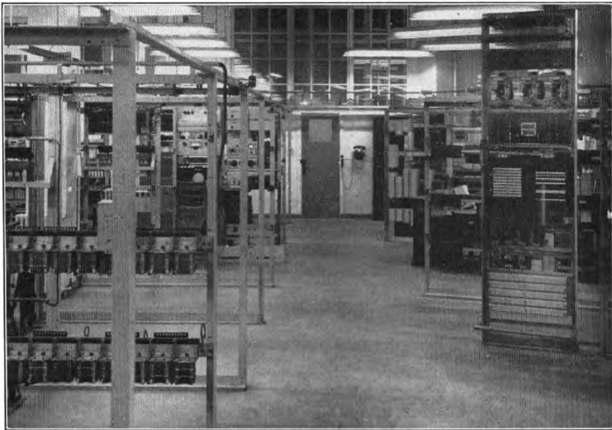
FIG. 2.—PART OF THE MAIN TESTING LABORATORY.
