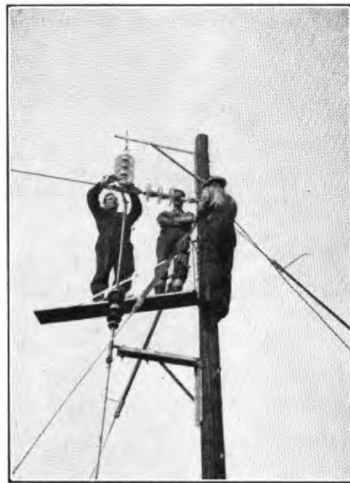
FIG. 3.—HEAD OF POLE A2, FITTED WITH CONDUCTOR RELEASING GEAR.
