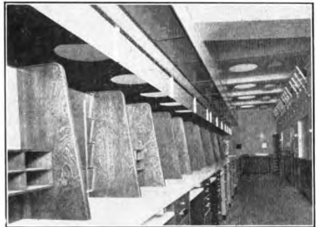
THE COUNTER LIGHTING INSTALLATION.
