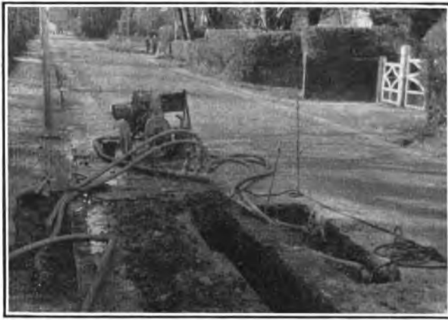
3-IN. SUCTION PUMP IN USE FOR DEWATERING.
