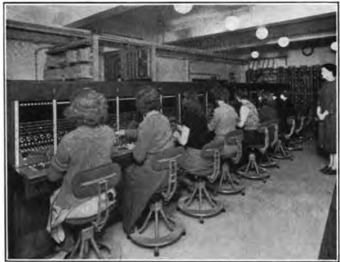
FIG. 3.—THE ADMINISTRATION SWITCHBOARD.
