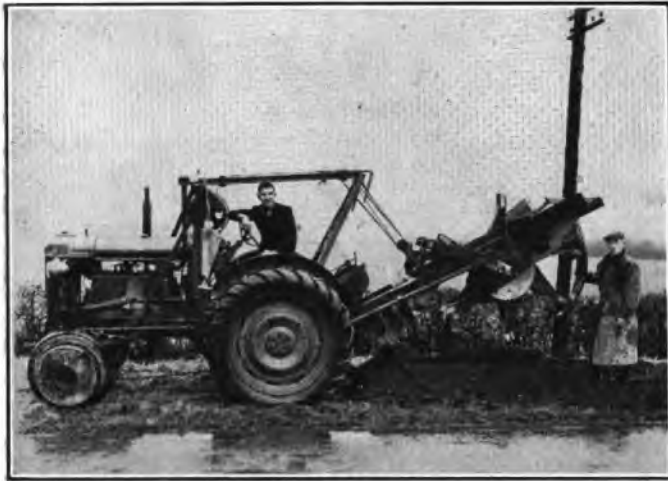
THE TRENCHING MACHINE WITH DIGGING ROTOR RAISED CLEAR OF TRENCH.
