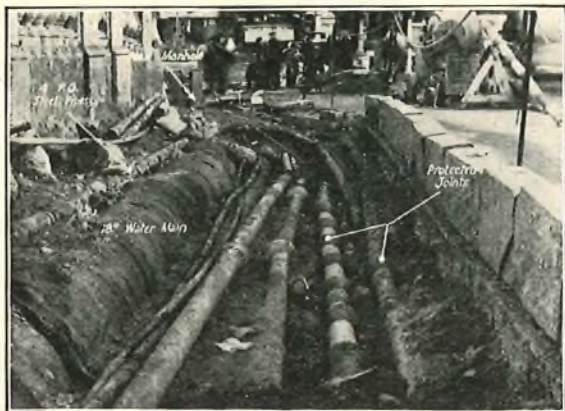
EXPOSED PLANT, INDICATING PROTECTION.
