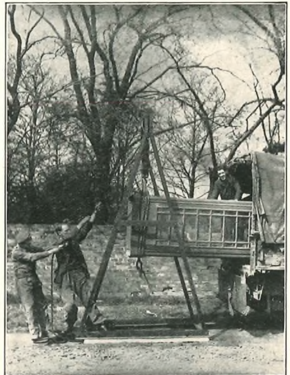
KIOSK LOADING OPERATION.
