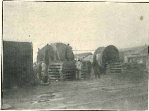
RE-DRUMMING CABLE AT PEMBROKE DOCK.
