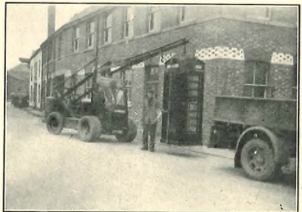
MOBILE CRANE IN USE FOR PLACING KIOSK.
