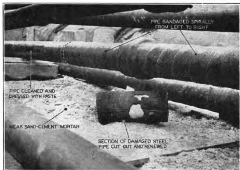
FIG. 4.—P.O. PIPE UNDER TREATMENT.
