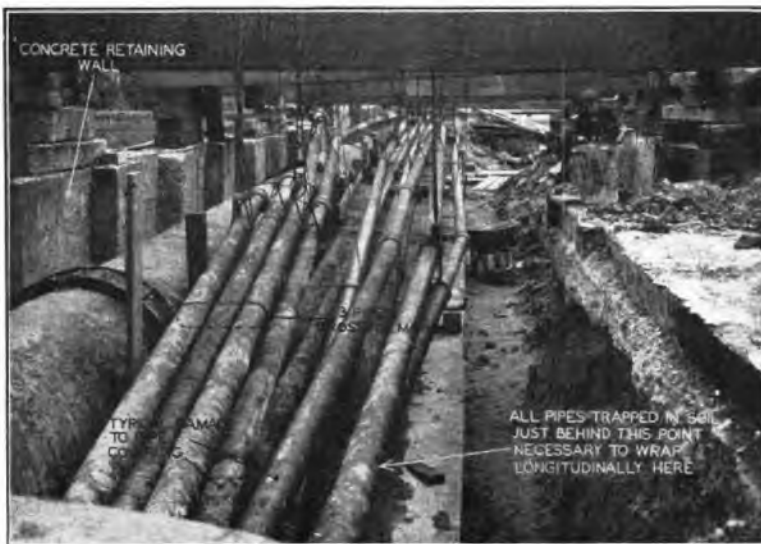
FIG. 3.—VIEW LOOKING EAST SHOWING RETAINING WALL.
