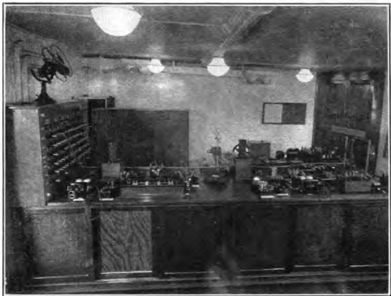
FIG. 10.—CABLE TESTING ROOM.
