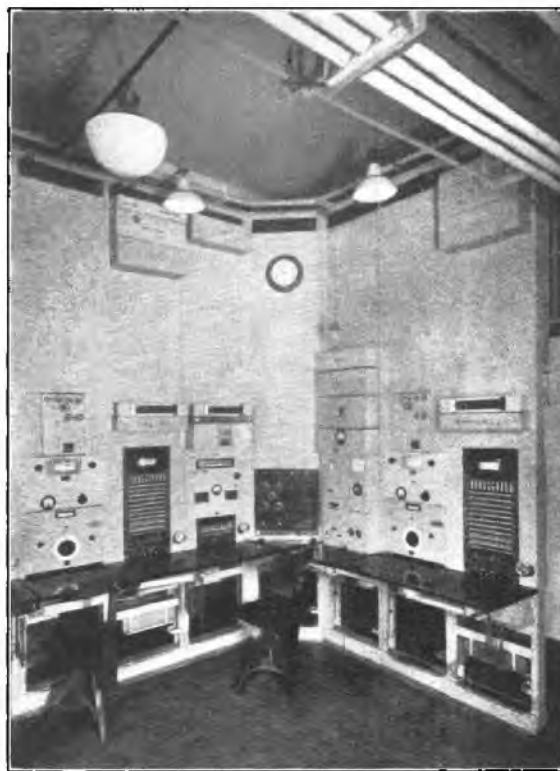
FIG. 3.—CORNER OF INLAND TRANSMISSION TESTING ROOM.
