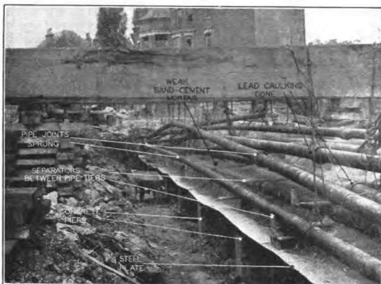
FIG. 5.—RECONDITIONING OF PIPES AT ADVANCED STAGE.
