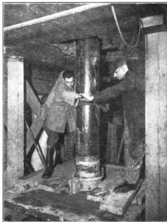
FIG. 2.—SCREWING IN A SECTION OF BORE TUBE.
