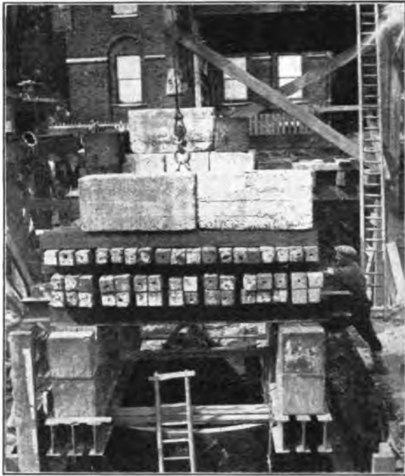
FIG. 5.—CYLINDER SINKING UNDER LOAD.
