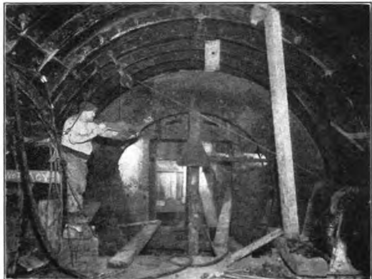
FIG. 6.—"GREATHEAD" SHIELD BEING ERECTED.
