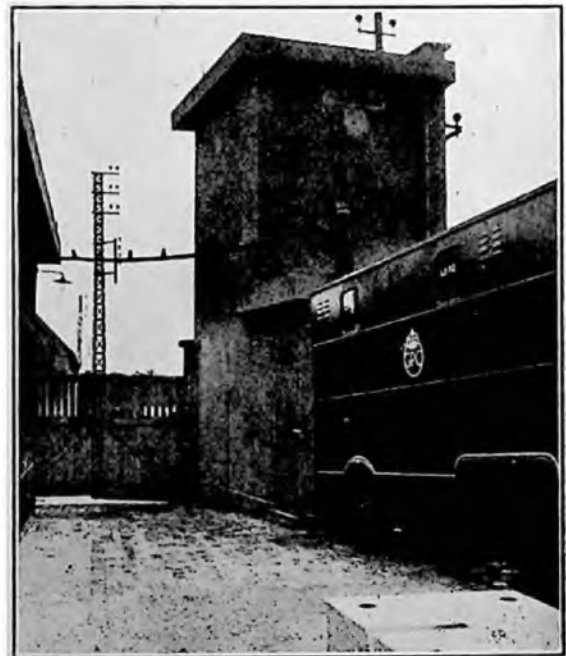
FIG. 7.—MOBILE CARRIER REPEATER STATION IN USE AT TILQUES.
