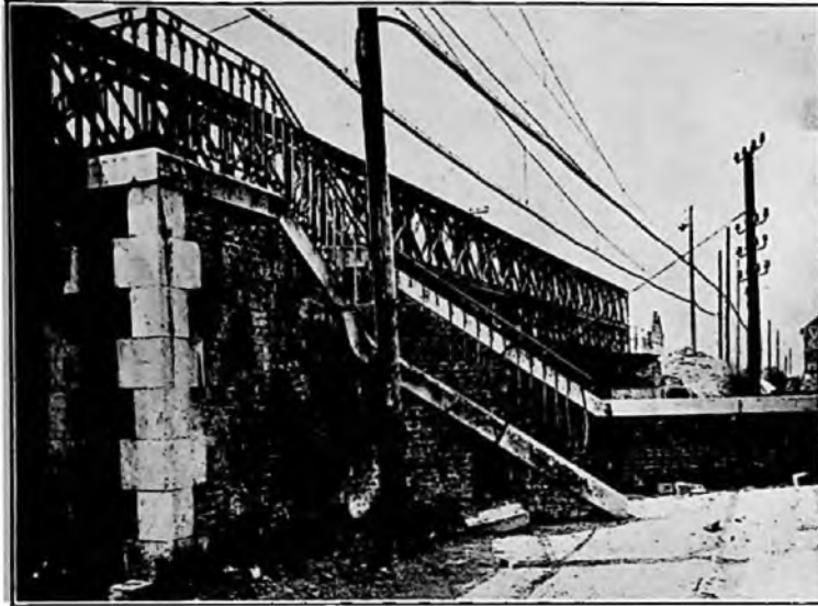
FIG. 2.—AERIAL SECTION OF BALANCED PAIR CABLE BY BAILEY BRIDGE OVER RAILWAY AT CALAIS.
