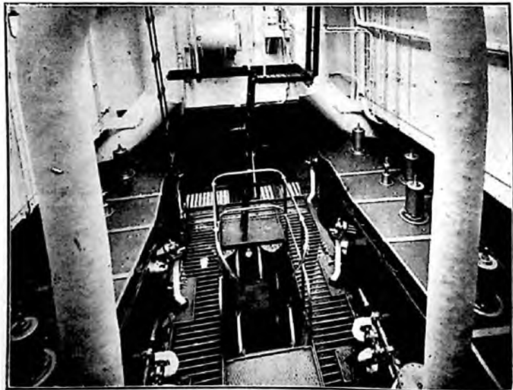
FIG. 6.—H.M.T.S. "IRIS." ENGINE ROOM (LOOKING AFT).
