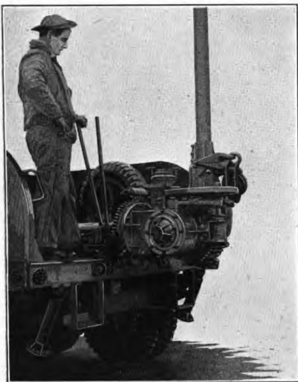
FIG. 1.—EARTH BORING MACHINE
