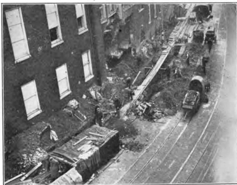
FIG. 6. BRIDGE CARRYING INTERRUPTION CABLE OVER BOMB CRATER.
