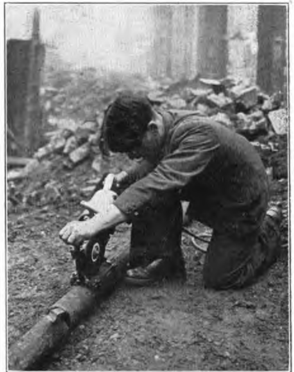
FIG. 2.—"SKILSAW" CUTTING STEEL PIPE.
