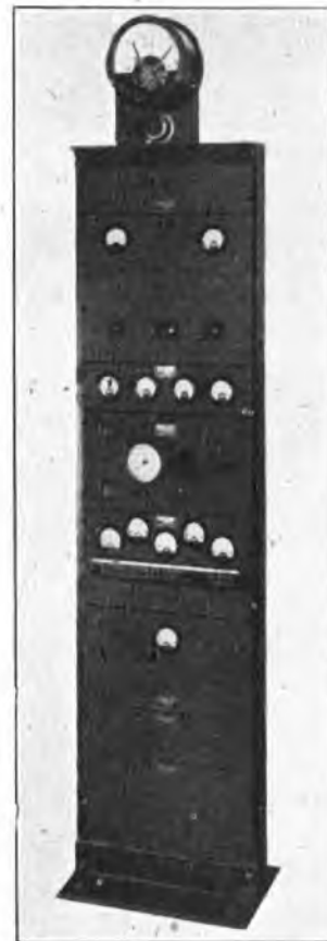
FIG. 3.—CONTROL BAY FOR FORK A.
