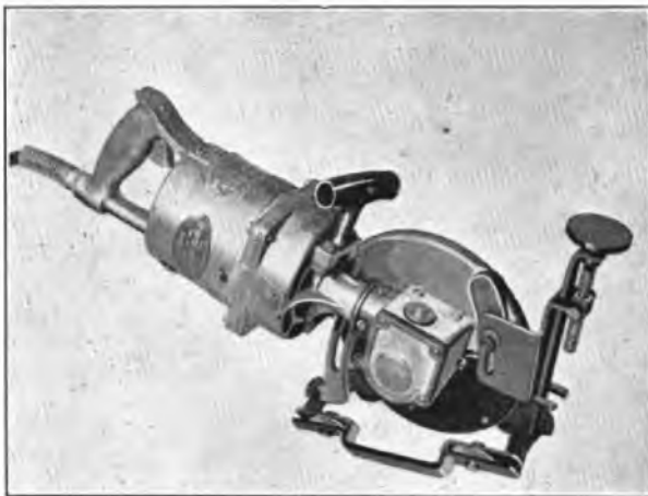
FIG. 1.—"SKILSAW" AND WHEELED CARRIER.
