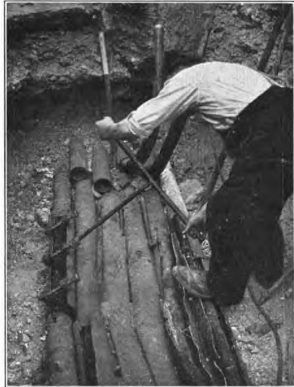
FIG. 4.—USE OF THE SCREW CLAWS.
