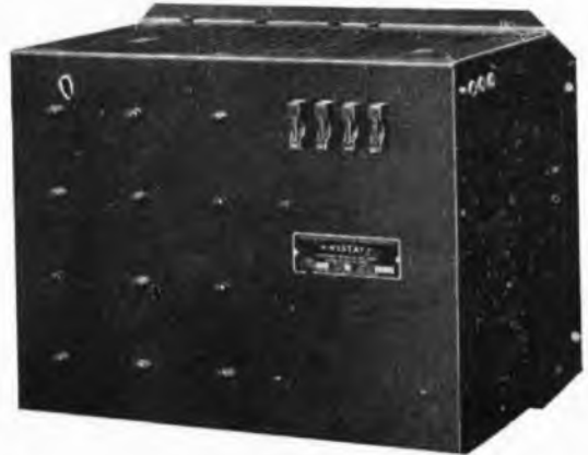
600 watt "Westat." Output 50.54 volts 12 amps.
