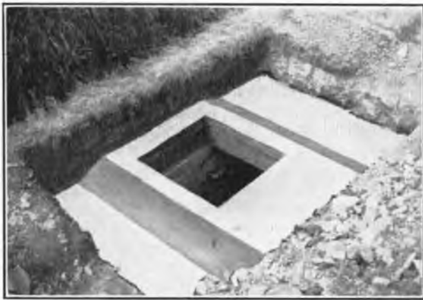
FIG. 5.—ROOF TOP SHOWING SPADE FINISH.
