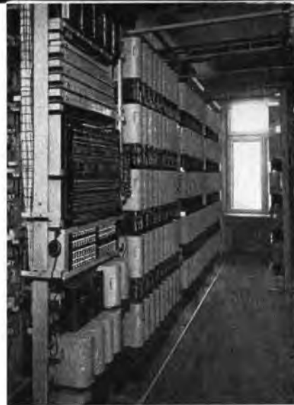
The illustrations show interior views of typical Strowger Automatic Telephone Exchanges in operation in various parts of the world.
