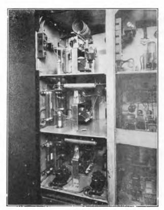
Fig. 3.—Crystal Frequency Amplifiers and Frequency Doubling Stages.
