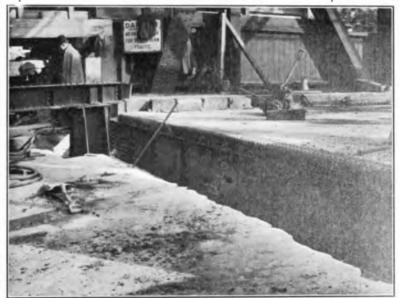
FIG. 7.—LEVEL OF BRIDGE SURFACE BEING RAISED.
