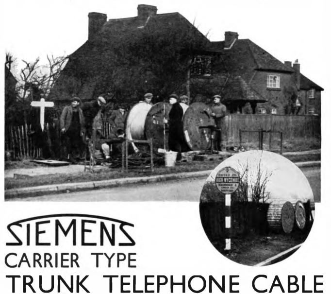
Two cables each 63 miles in length, are laid in the same duct. 24 pairs, 40 lbs., air-space, star quad. Designed to operate up to 60 kilocycles per second.
