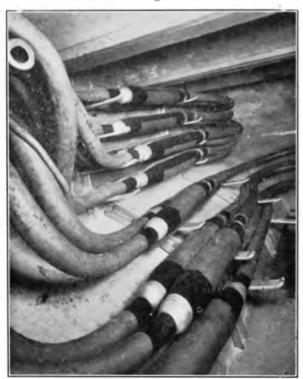
Fig. 5.—Completed Joints in Manhole Outside Brettenham House.
