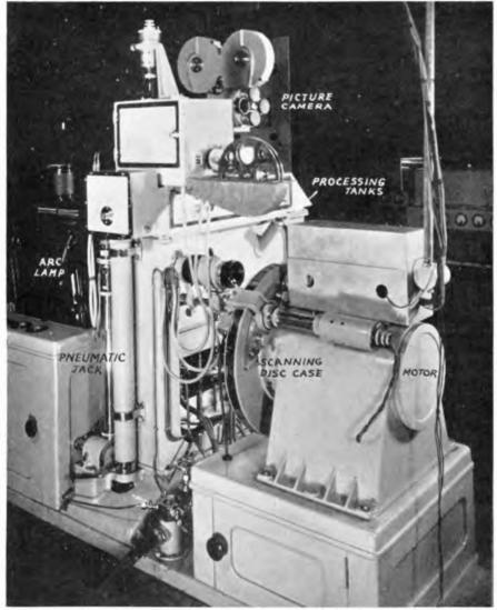
FIG. 8 .- BAIRD INTERMEDIATE FILM TRANSMITTER,
