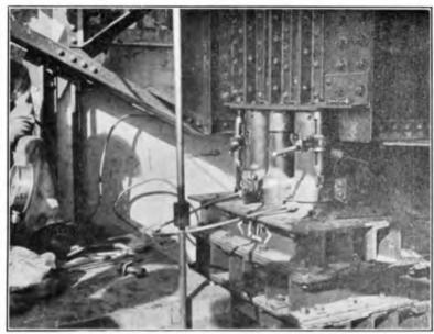
FIG. 6.—BANK OF HYDRAULIC LIFTING JACKS.
