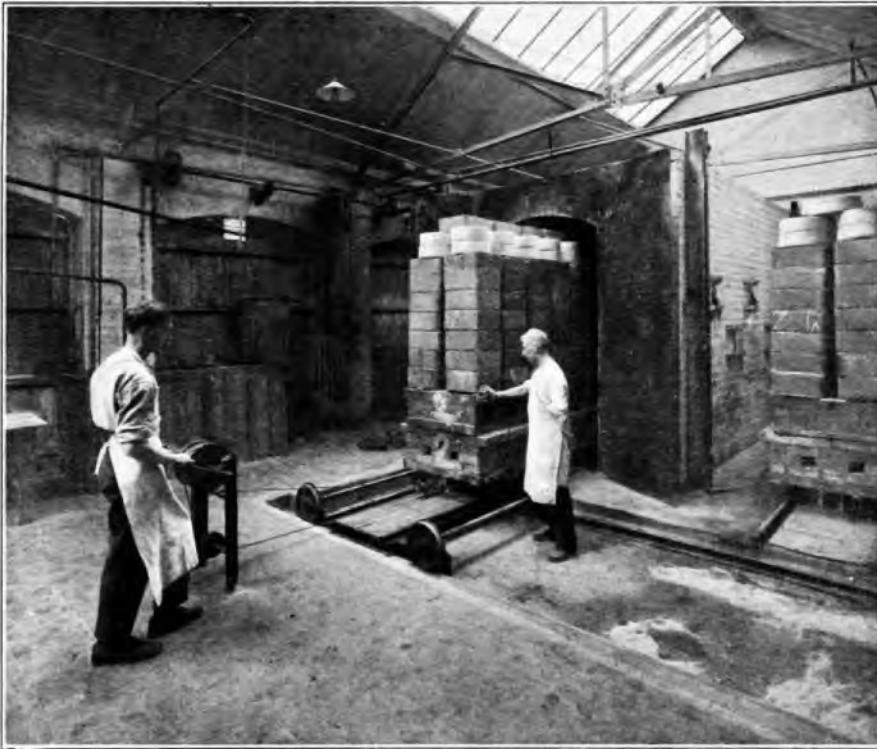
FIG. 4.—EXIT END OF TRUCK OVEN.
