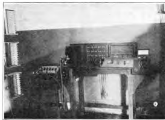
FIG. 5.—TRUNK TEST DESK.
