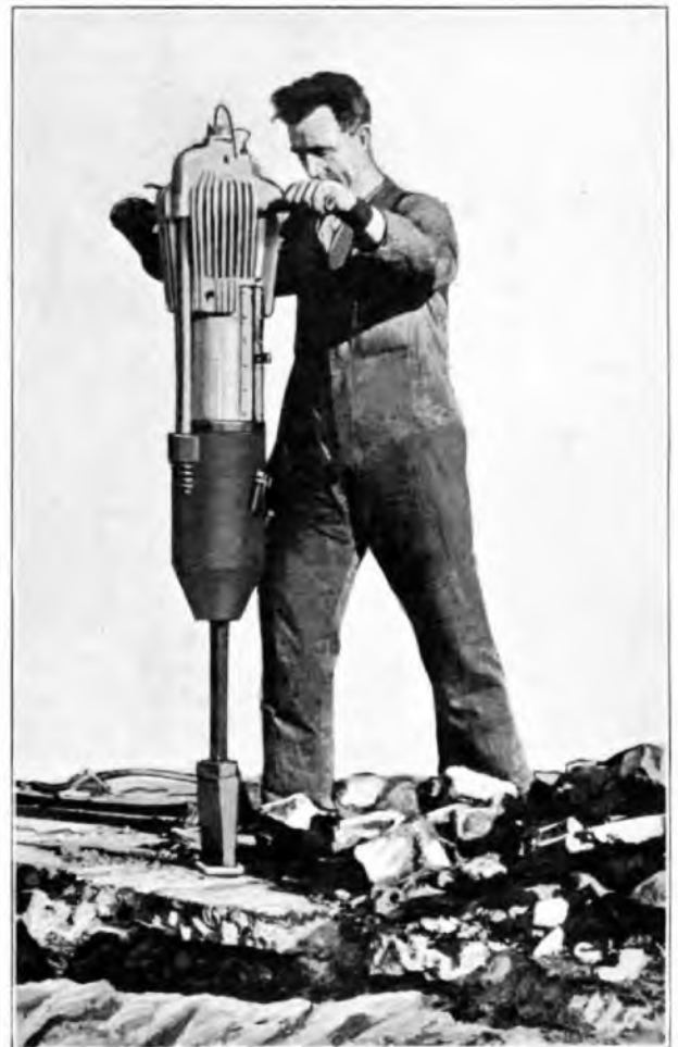
FIG. 3.—CONCRETE BREAKING ATTACHMENT ON "JOHNSON" RAMMER.
