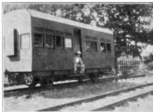
FIG. 8.—RAILWAY COACH ALLOTTED FOR MAINTENANCE.
