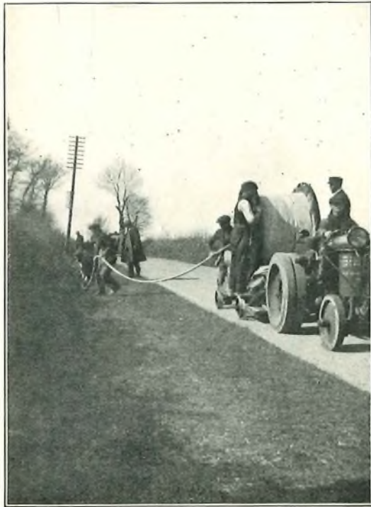
FIG. 4.—LIFTING CABLE INTO POSITION.
