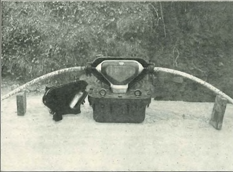
FIG. 2.—BURIED LOADING POT.
