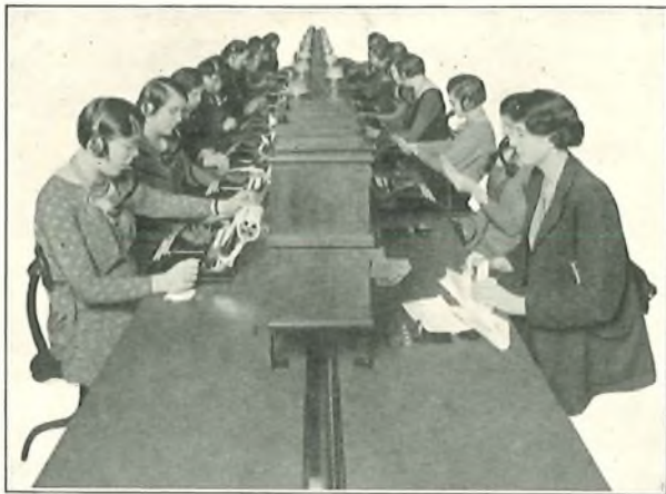
FIG. 1.—END VIEW OF A TYPICAL TELEPHONE-TELEGRAM SUITE, SHOWING V-BELT CONVEYOR.
