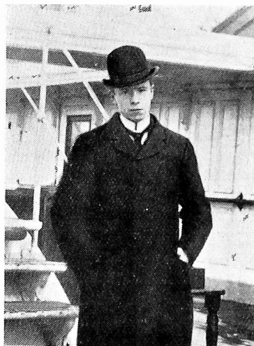
A photograph of the late Mr. F. S. Stacey taken in 1900 on board the Belgian mail steamer "Princess Clementine," the first cross-Channel steamer to be fitted with Marconi equipment.
