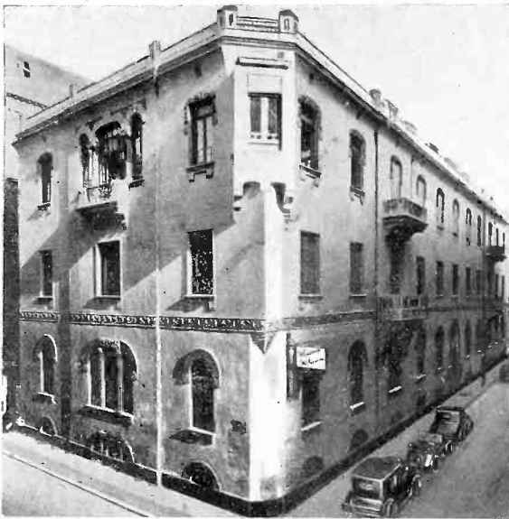
Radio House, Cairo: Headquarters of Egyptian State Broadcasting.
