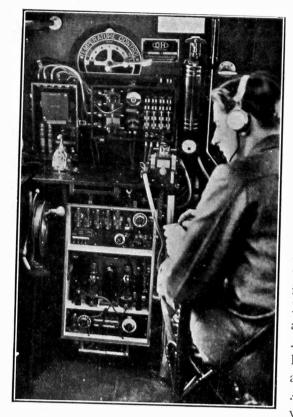
Marconi A.D. 6 Aircraft set fitted in Imperial Airways passenger machine.
