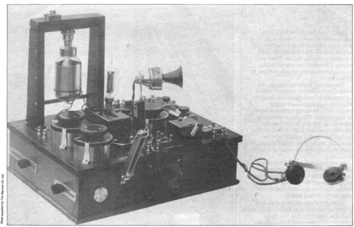
Set used by Marconi during telephone experiments between vessels at anchor 10 kilometres apart in Italy 1914.
