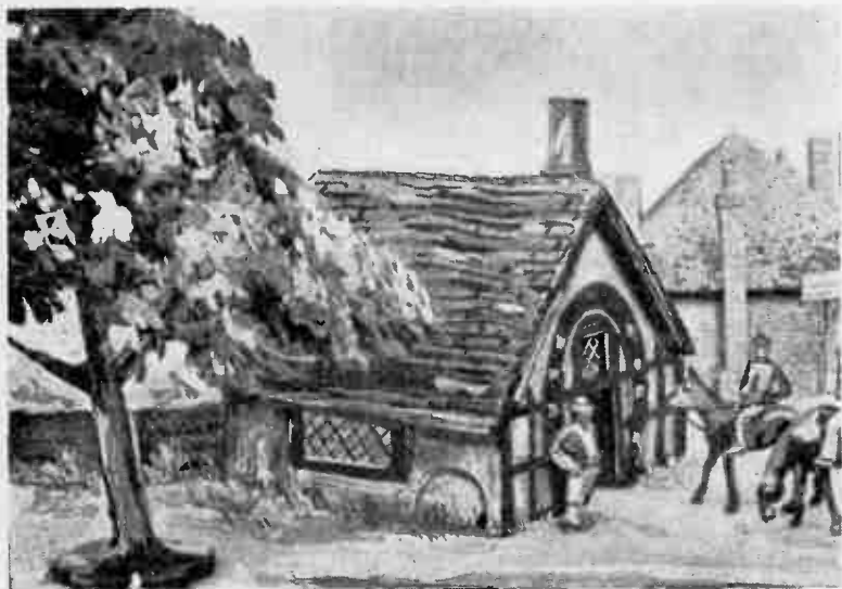
The completed smithy and tree
