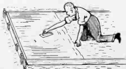
Fig. 5—Using the float on the work
