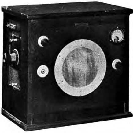
Fig 8 The original Rice Kellogg moving-coil loudspeaker. The field coil power supply and driving amplifier are built in (circa 1925).
