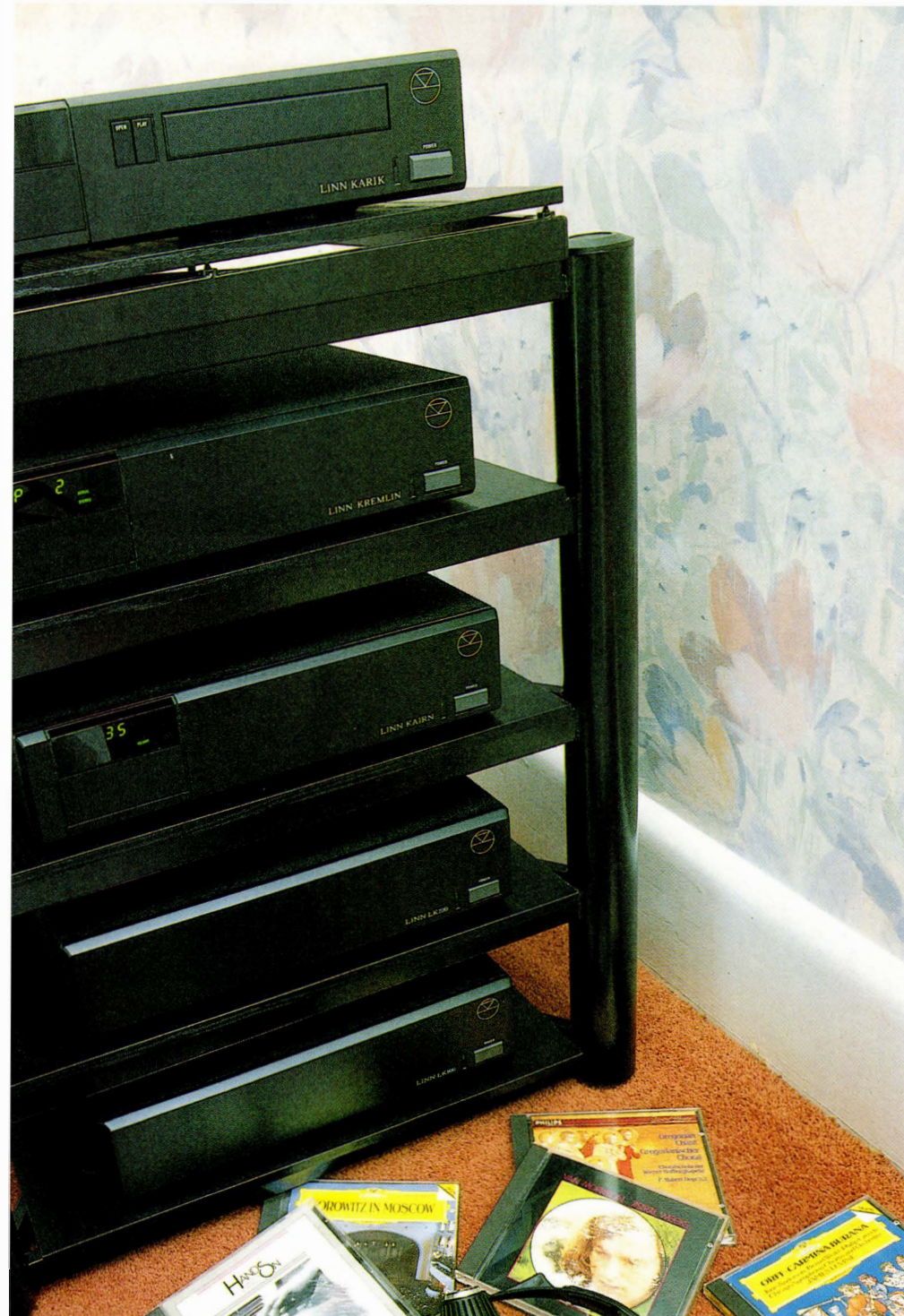
The Linn crowd. Michael's professionally installed Linn electronics sit proud on Tripod's equipment stand.
