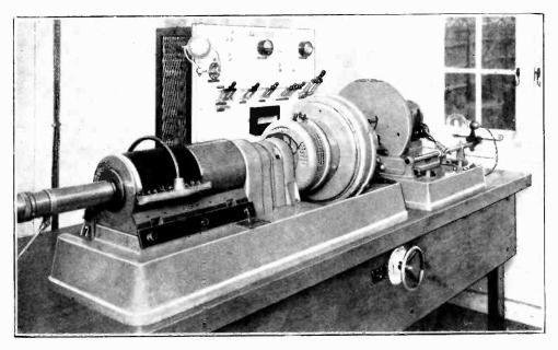
Picture transmitting equipment. The tube on the left carries the dispersed light from the image to the photoelectric cell.
