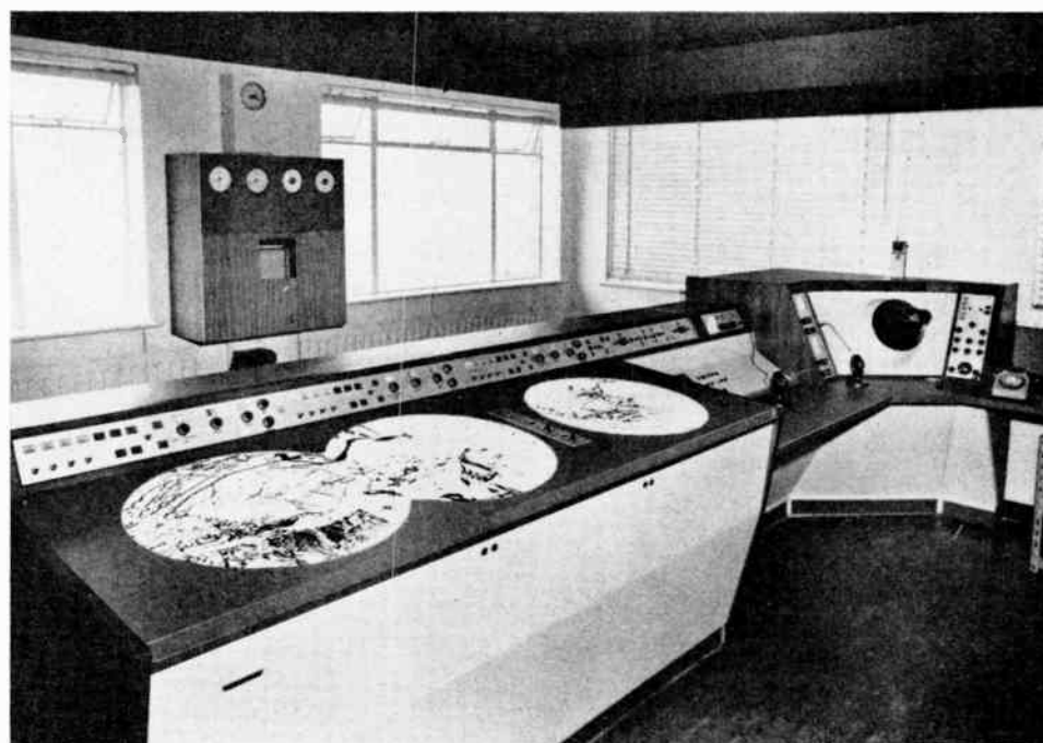
Fig. 8. Control room, Teesport.
