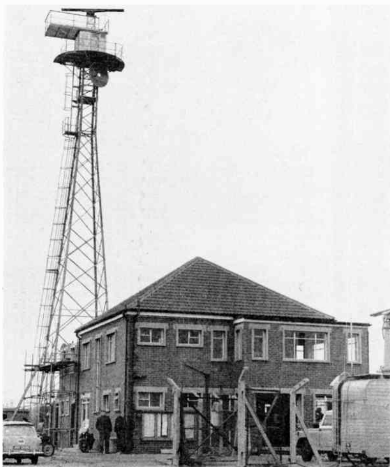
Fig. 7. Control station and antenna mast, Teesport.
